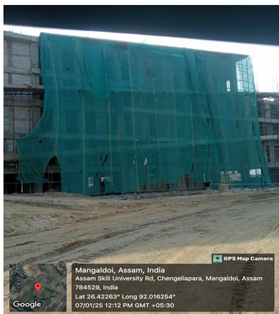
The green-net provided at working building area to minimize dust emission
