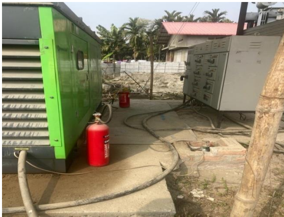
Fire extinguishers and rubber mat provided near DG
