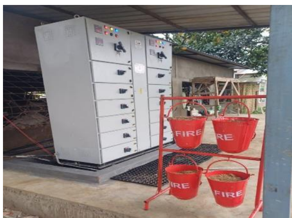
Fire buckets and rubber mats placed near panels
