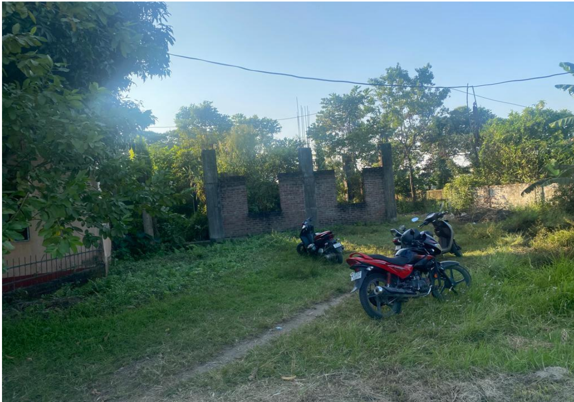
Front View of Interim Campus at ITI Guwahati
