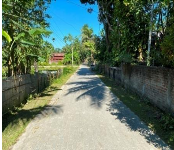
View of Access Road Connecting Site with NH
