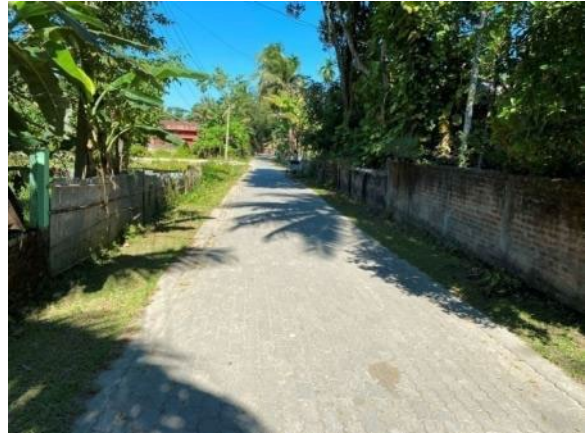
Another View of Access Road
