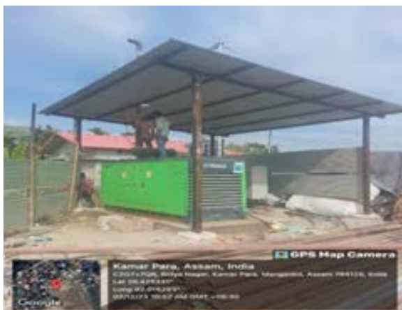
DG set stack height installed as per CPCB requirement.
