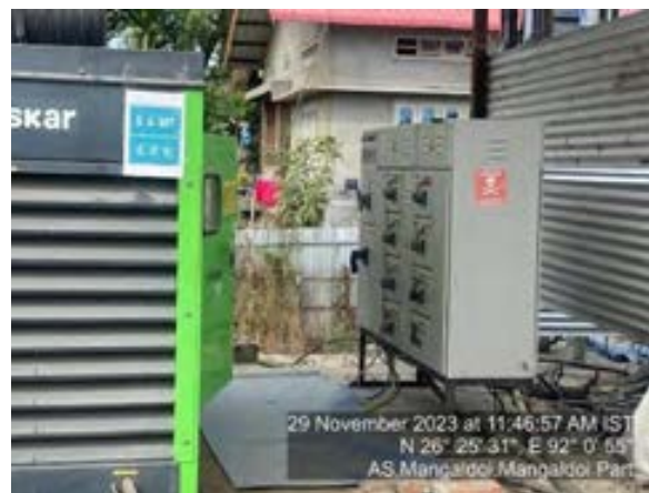
Electrical panel provided with rubber mat.
